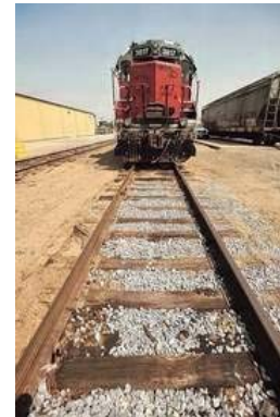
San Joaquin Valley Railroad in Exeter at Palm Street between North G and North F streets. (Steve R. Fujimoto)
